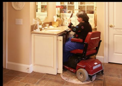
Finished flooring under sink
